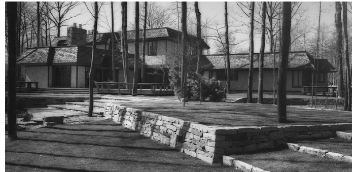
Eleanore K. Pettersen Residence and Studio: courtyard and exterior. Saddle River Road, N.J.
