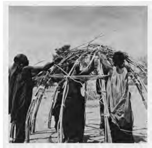
Fulbe women erecting a matframe tent, north of Bamako, Mali. Photo from Hatumere: Islamic Design in West Africa by Dr. Labelle Prussin, 1986.
