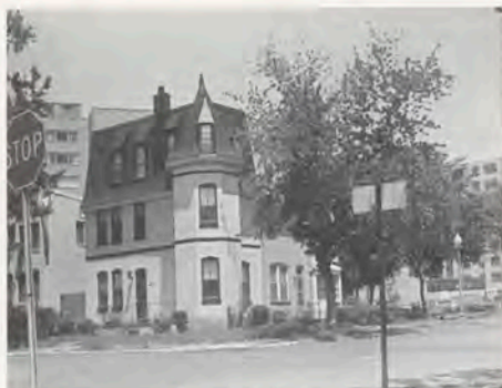
Melita's house in Foggy Bottom, an historic restoration among Washington D.C. institutions and modern buildings.
